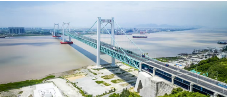
The Wenzhou Oujiang Beikou Bridge Project received the NCE International Bridge Award
