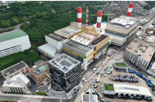
Macao Waste Incineration Center Phase III Expansion
