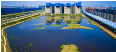
The First Harbor Engineering Group assisted in establishing an ecological circulation water system at Huanghua Port, achieving zero wastewater discharge and full reuse of outlet water in the port area
