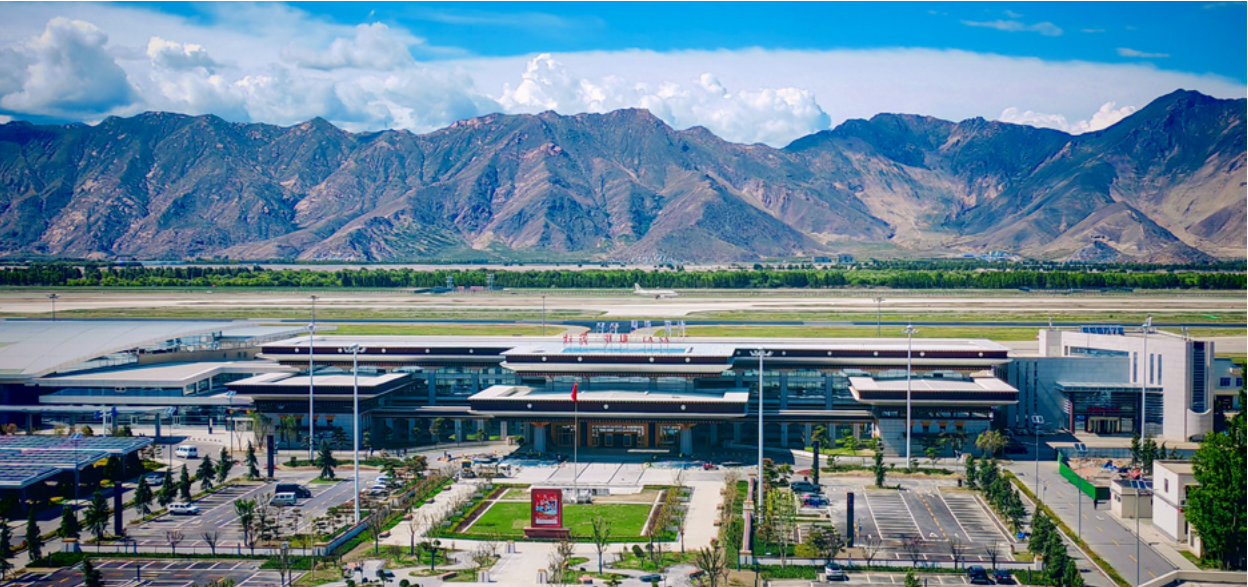
Lhasa Gongga Airport Expansion Project – Bid Section 2
