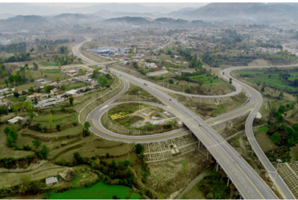
Pakistan's Karakoram Highway Phase II Project
