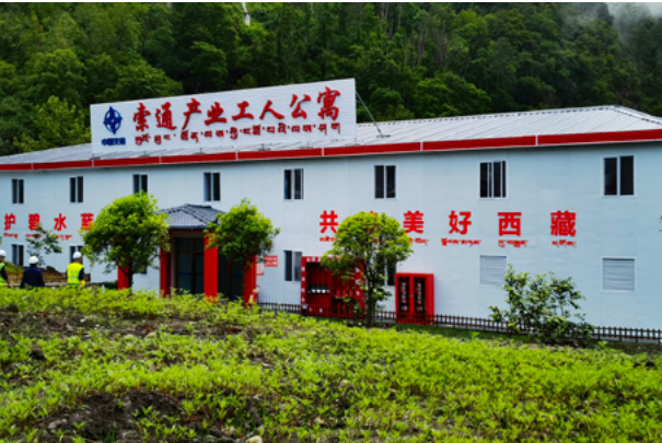
Sotown Industrial Workers' Apartment
