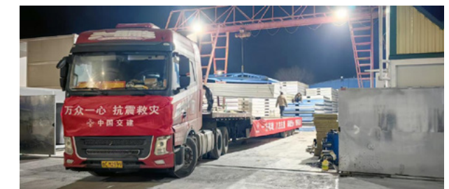
The first batch of containerized modular houses, overseen by the First Highway Engineering Group, arrives at the resettlement site in Lhaze County
