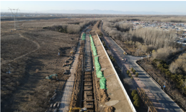
Yongding River Project Construction Site
