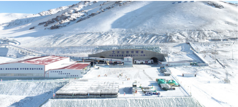
Tianshan Shengli Tunnel
