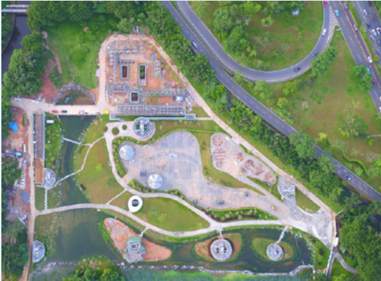
The Phase I project of the Shenzhen Honghu Water Purification Plant by the Southwest Institute, known as the "Shenzhen He Water Culture Science Popularization Base," received the 2024 Global Project Excellence Award (Silver) in the ultra-large/large infrastructure category, marking the first IPMA award in China's water industry to date
