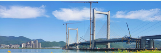
The Meishan Waterway Bridge of the Liheng Expressway Project in Ningbo, Zhejiang
