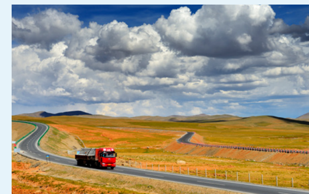
High-Altitude Qinghai-Xizang Permafrost Highway Construction and Maintenance Technology
