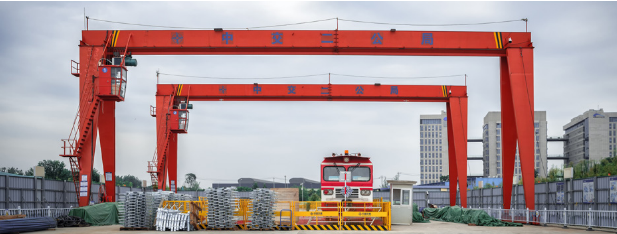
Standardized management at the Chengdu Metro Line 30 track laying base
