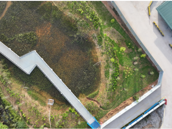
The CR205 King Albert Park MRT Station interchange station project of Singapore's second-phase Cross-Island MRT Line underwent ecological environment relocation in its marsh area
