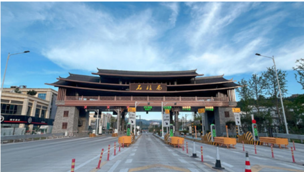
CCCC Asset Management's Shizhu West Smart Toll Station Renovation
