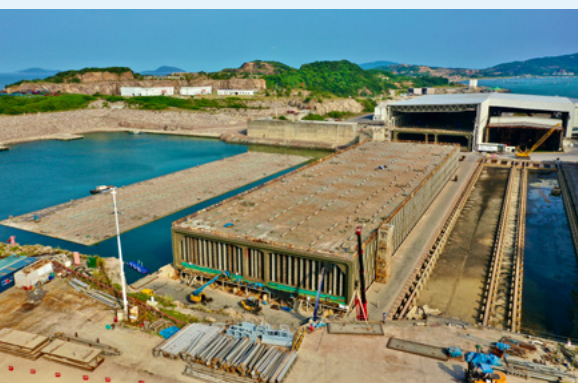
Immersed Tube Tunnel Construction Technology
