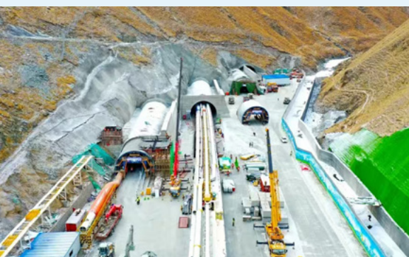
Ultra-Long Tunnel Construction Technology
