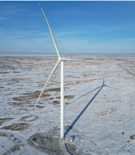
Jilin Da'an Wind Power Project
