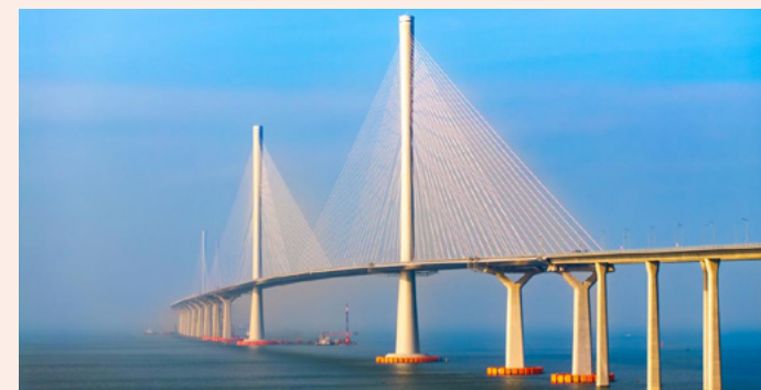
A major cross-sea project in the Guangdong-Hong Kong-Macao Greater Bay Area: the Huangmao Sea Channel Bridge
