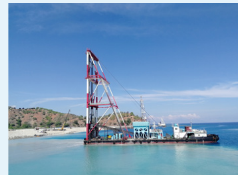
Intelligent Offshore Vibroflotation Stone Column Piling Barge
