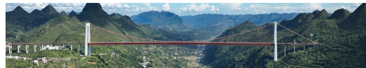
Baling River Bridge
