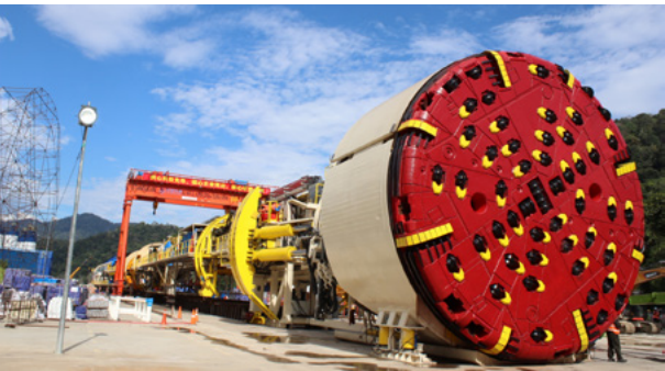
Malaysia East Coast Rail Link Project
