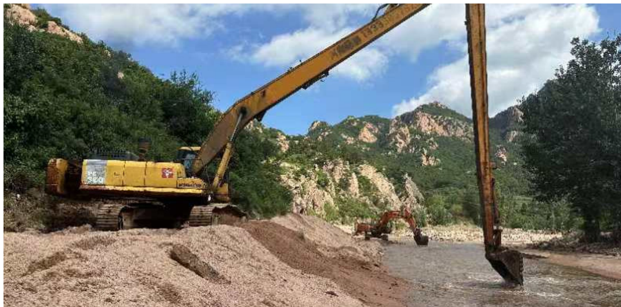
CCCC First Harbor Engineering Company rushes to aid in the Huludao flood disaster
