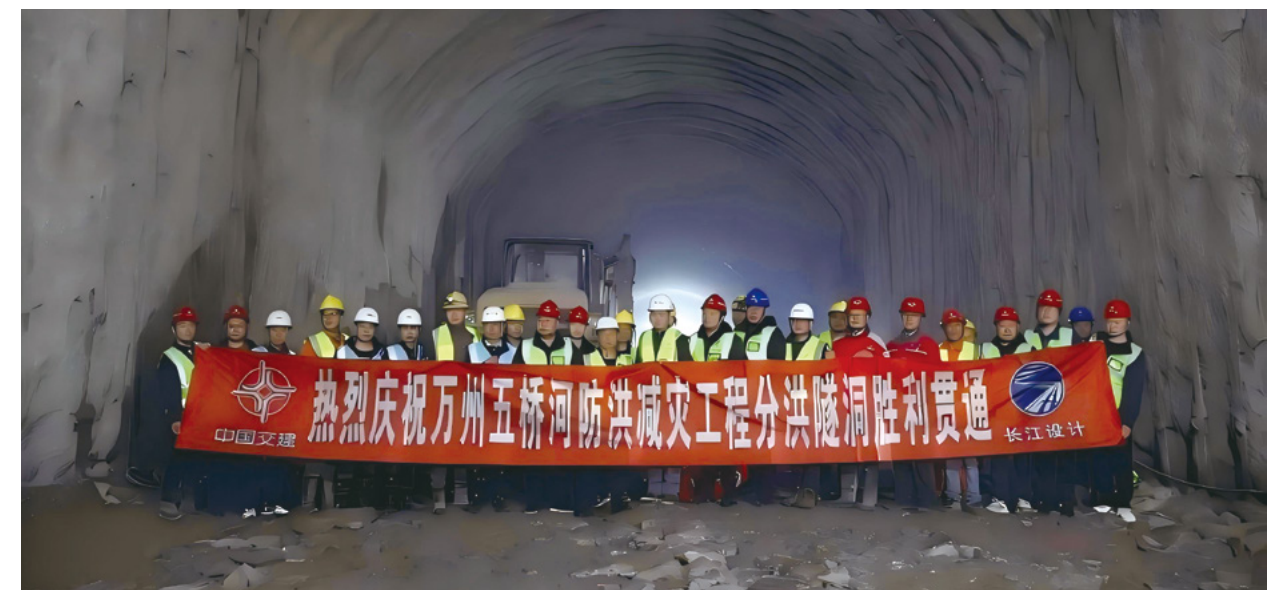
The diversion tunnel of the Wuqiao River Flood Control and Disaster Reduction Project in Wanzhou, Chongqing, has been completed
