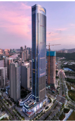
CCCC Huitong Hengqin Plaza Project
