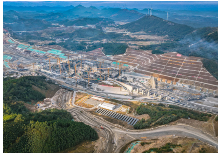
Panoramic View of the Pinglu Canal Foundation Pit
