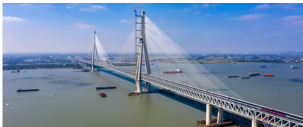
The Changtai Yangtze River Bridge was closed with "millimeter-level" precision
