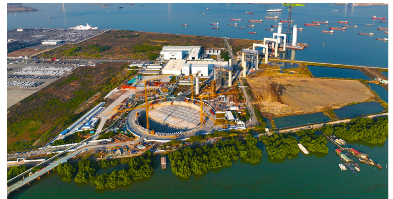
The west anchorage of the Shiziyang Passage project bridge has completed core filling construction
