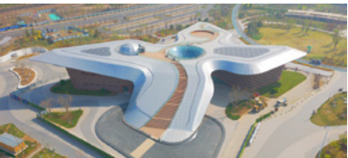
CCCC Investment's Tianjin Design Capital Project Ecological Science and Technology Pavilion achieved an overall building energy saving rate of 64% and a building envelope energy saving rate of 51%, and obtained a near zero-energy building design stage certification from the China Association of Building Energy Efficiency.
