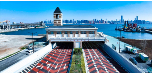
Dalian Bay Undersea Tunnel received the Best Project Award in the Bridge and Tunnel category
