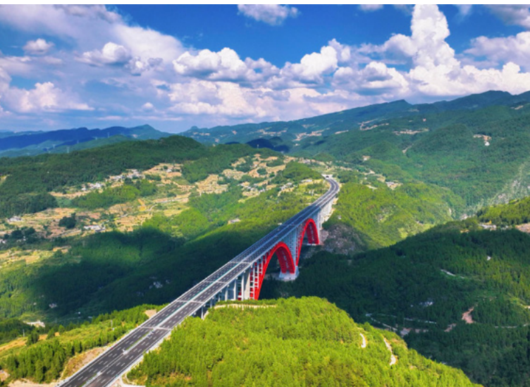
The Shuangbao Bridge, with the world's largest dual-cable-stayed span featuring independent towers and unprecedented construction weight for such structures, set a global record
