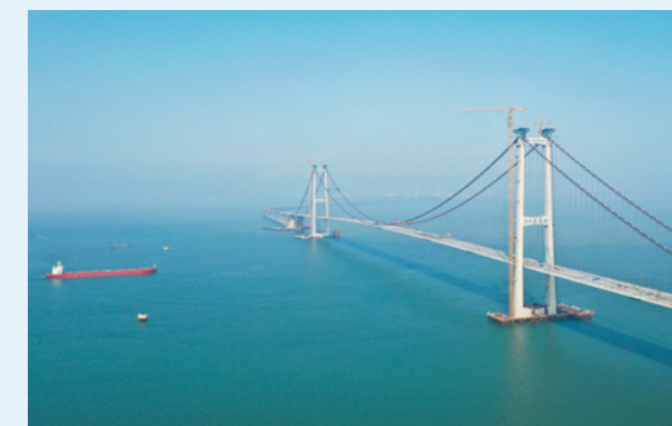
Super-Large Span Bridge Construction Technology
