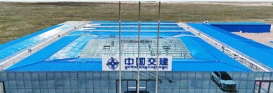
The Nagqu project in Xizang built a green and smart project site
