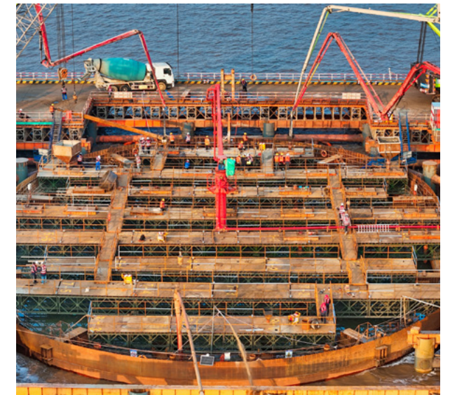
At the Hangzhou Bay Cross-Sea Railway Bridge, the first main pier cap at the south channel bridge has been capped
