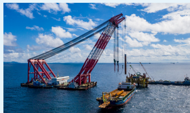
Offshore Wind Power Foundation Construction and Turbine Installation Technology
