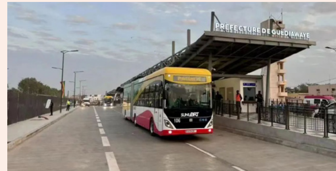
Senegal's first Bus Rapid Transit system: the Dakar BRT Project
