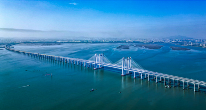
Fuzhou-Xiamen High-Speed Railway 's Quanzhou Bay Cross-Sea Bridge received the Theodore Cooper Award (Railway Bridge Award) and the FIDIC Excellence Award
