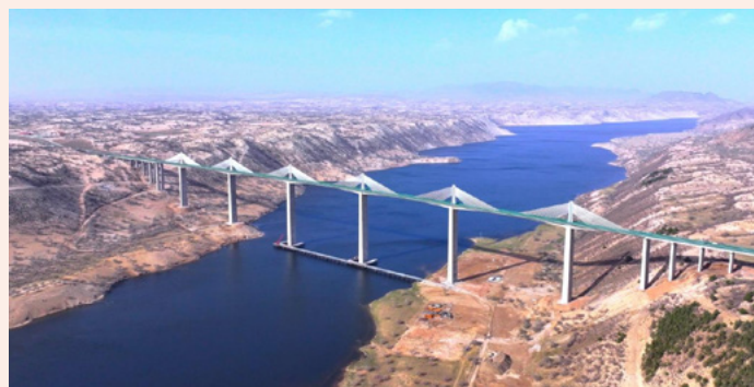
The world's first bridge built in a wind-blown sand gorge and the world's highest, longest-span PC beam multi-tower cable-stayed bridge: the Xilamulun Grand Bridge in Inner Mongolia
