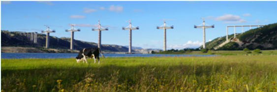
The Xilamulun Bridge in Chifeng, Inner Mongolia
