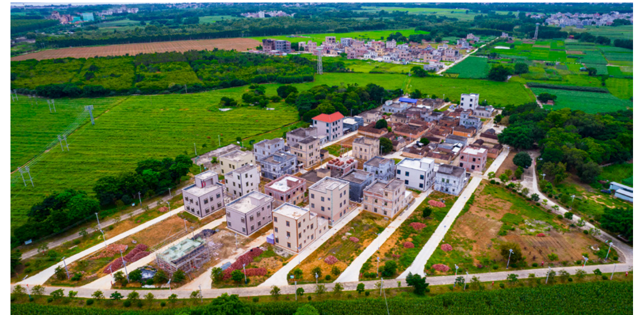
Projects in progress include the road hardening and lighting project for Neijiao Village in Jiepao Town, Suixi County
