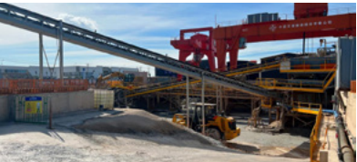
The Third Harbor Engineering Institute's Xiamen Metro Line 4 project achieved the reuse of inorganic raw materials and water resources
