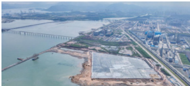
The supporting project (Section One) of the Fourth Harbor Engineering's Huizhou Phase III Ethylene Project reduced earth and rock extraction by approximately 180,000 cubic meters, achieving resource recycling
