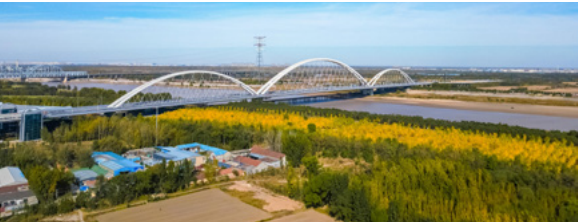
The Qilu Yellow River Bridge in Jinan– the longest bridge over the Yellow River and the inland highway bridge with the largest steel structure usage – was opened for operation
