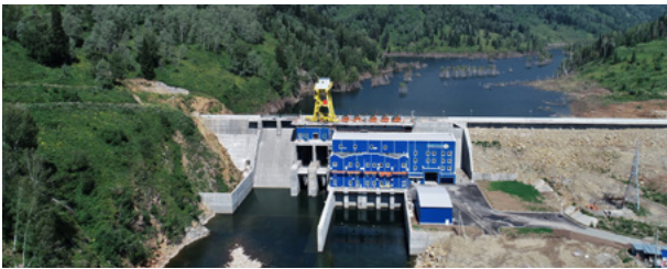
Turgusun Hydropower Station, Kazakhstan
