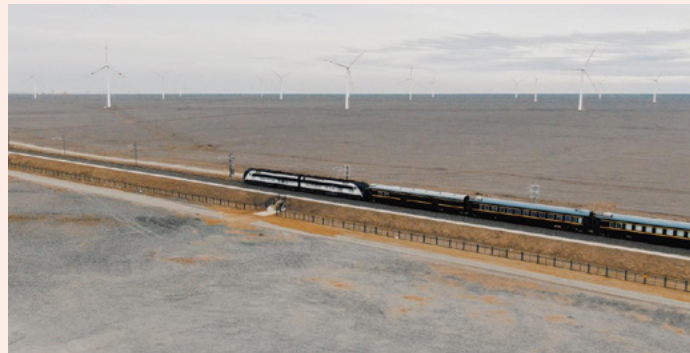
The first BOO-mode freight railway led and constructed by CCCG: the Jiangjunmiao-Naomaohu Railway in Xinjiang
