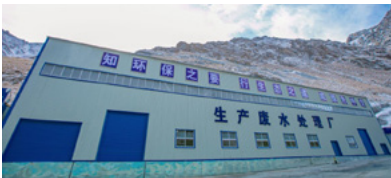
The General Contracting Subsidiary's Tianshan Shengli Tunnel project built 3 smart sewage treatment plants that process 17,500 cubic meters of wastewater daily, with all treated water used for construction production and dust suppression
